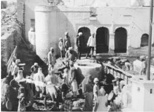
A view of the demolition work at the old Garhi Sahib Gurdwara where a new gurdwara in marble has come up in Chamkaur Sahib. — A file photograph
